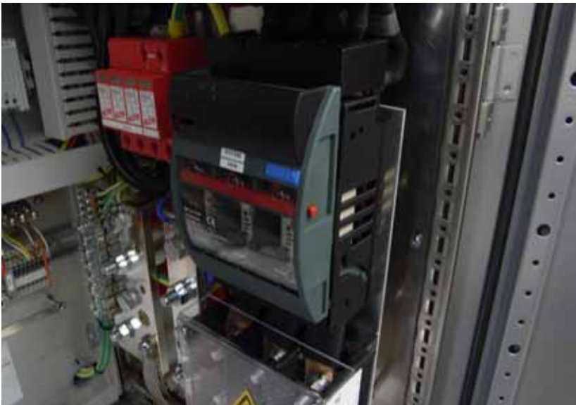
Figure 7.2: Different kind of AC grid connection terminals
