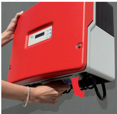
Step 1: Remove the ESS handle
