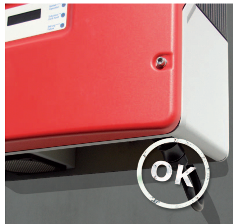
Finished: The inverter is isolated on the DC side.
